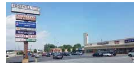
Commercial assets like the Edgehill Shopping Center on Route 13 in Dover are one of the many properties in Delaware that R&R provides property management services for.
