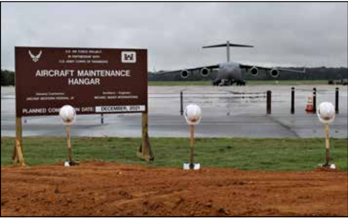
The Aircraft maintenance hangar was designed by Michael Baker International and will be built by Archer-Western.
