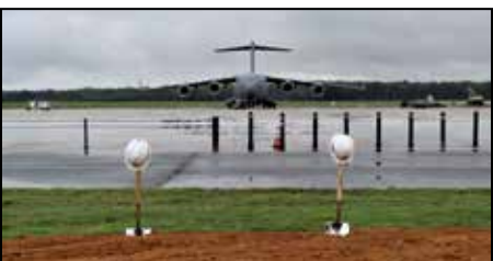
The C-5 and the C-17 will be completely enclosed in the new facility.
