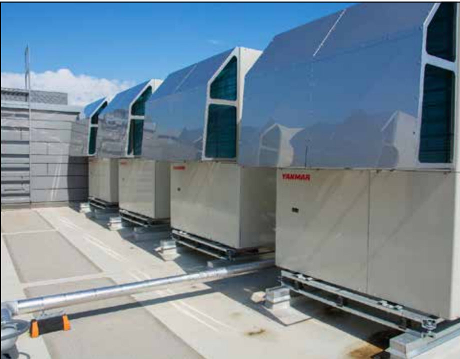
Gas Heat Pump units at the Chesapeake Utilities Corporation's Energy Lane Campus
