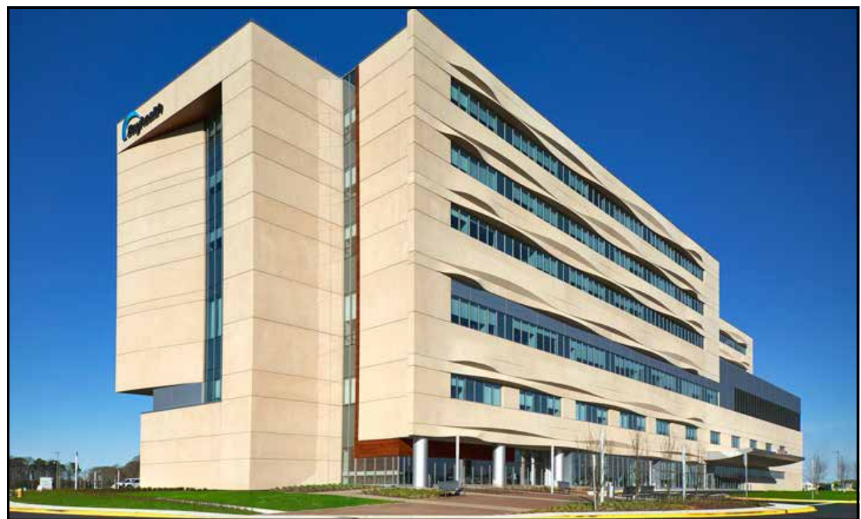
Bayhealth Hospital, Sussex Campus Inspection
